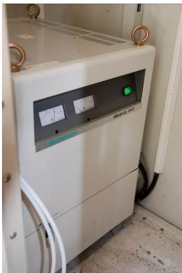
Photo 2.7-2 Noise cut transformer for power supply.
